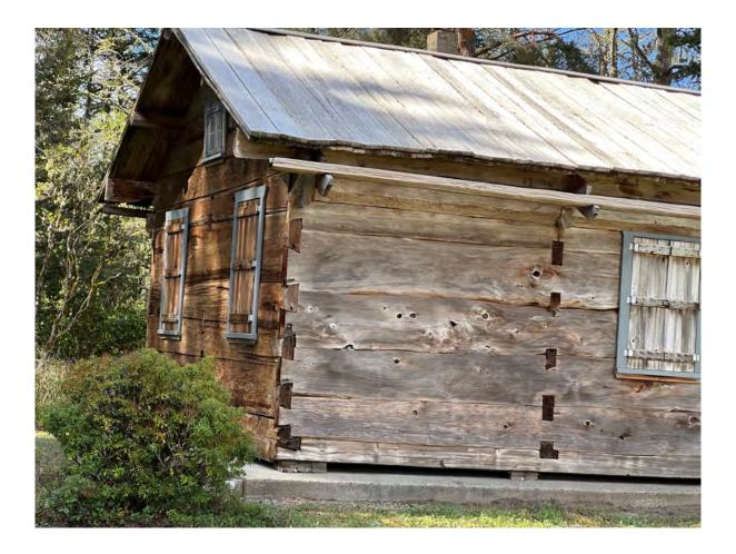
The Lindgren log home reconstructed at Cullaby Lake County Park was built by Finnish immigrants in the early 1900's. The logs are locked together at the corners and where the interior walls lock onto the exterior walls. These uniquely shaped "Dovetail" joints are cut at angles and sloped so moisture will flow out of the joint and away from the house. The house is behind a fenced area at the park and will be opened for visiting during summer weekends.
